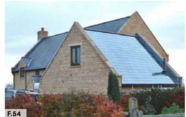
Figure 54: Positive example of a new build in which solar panels were integrated into the design from the onset
