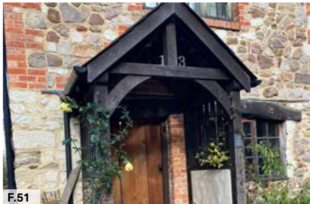
Figure 51: Detail of a building with rubble infilling, red brick dressing, and a timber gabled porch
