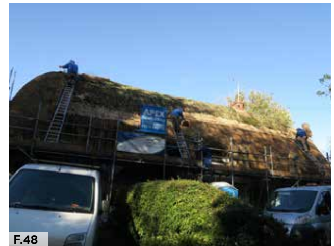
Figure 48: Renovation of a traditional thatched roof with "eyebrow" dormers
