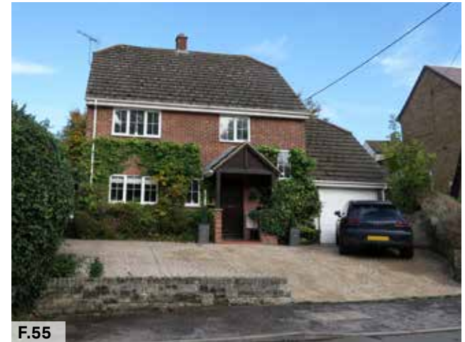
Figure 55: Photo of a front garden with impervious surfacing that could be replaced with permeable paving
