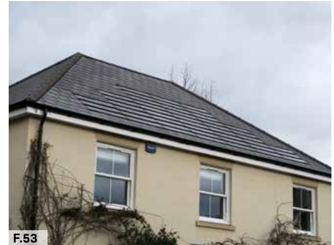
Figure 53: Photo of a building in Lingfield, Surrey with solar shingles successfully embedded into the slate roof
