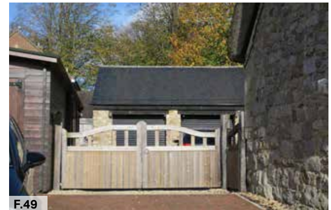
Figure 49: Modern back garage constructed with traditional local materials - rubble stone, slate tiles, and timber
