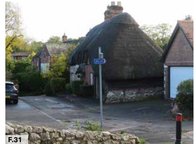
Figure 31: Photo of Slipper Lane showing a diversity of roof shapes and building layouts on the same frontage
