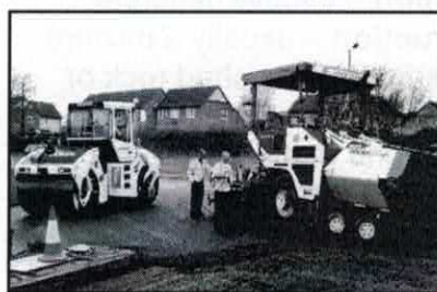
Conventional road surfacing process
