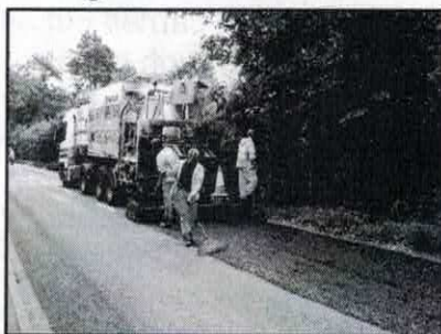
Microasphalt laying
